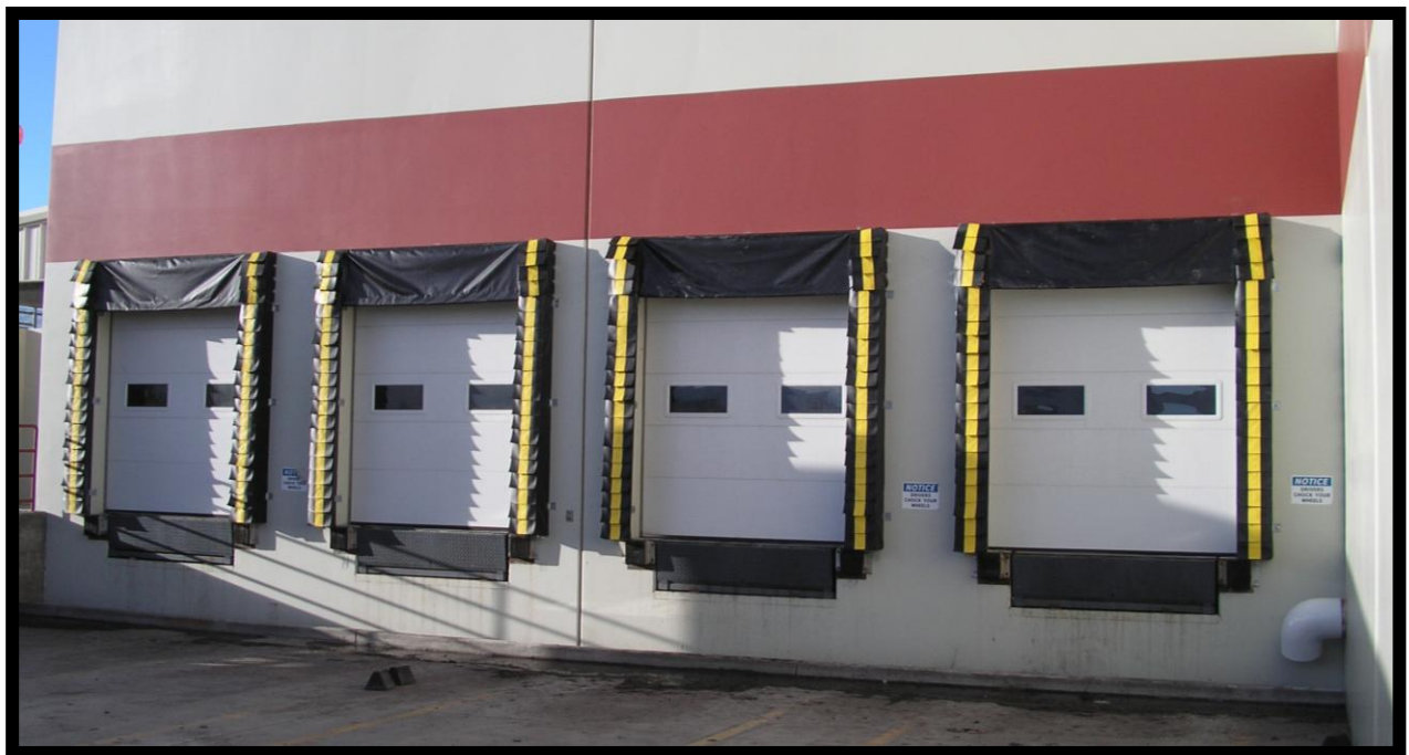
Dock Seals - After
