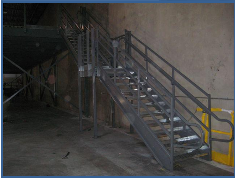
150 PSI Mezzanine with Extra Width Columns
