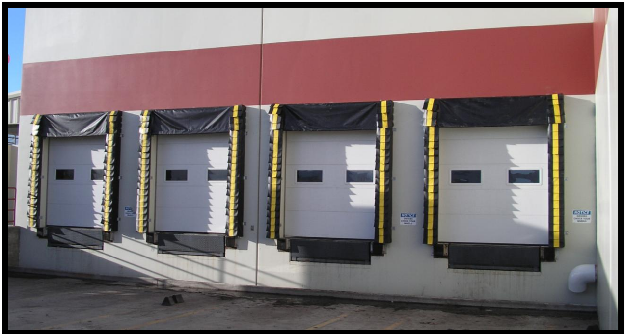
Dock Seals - After
