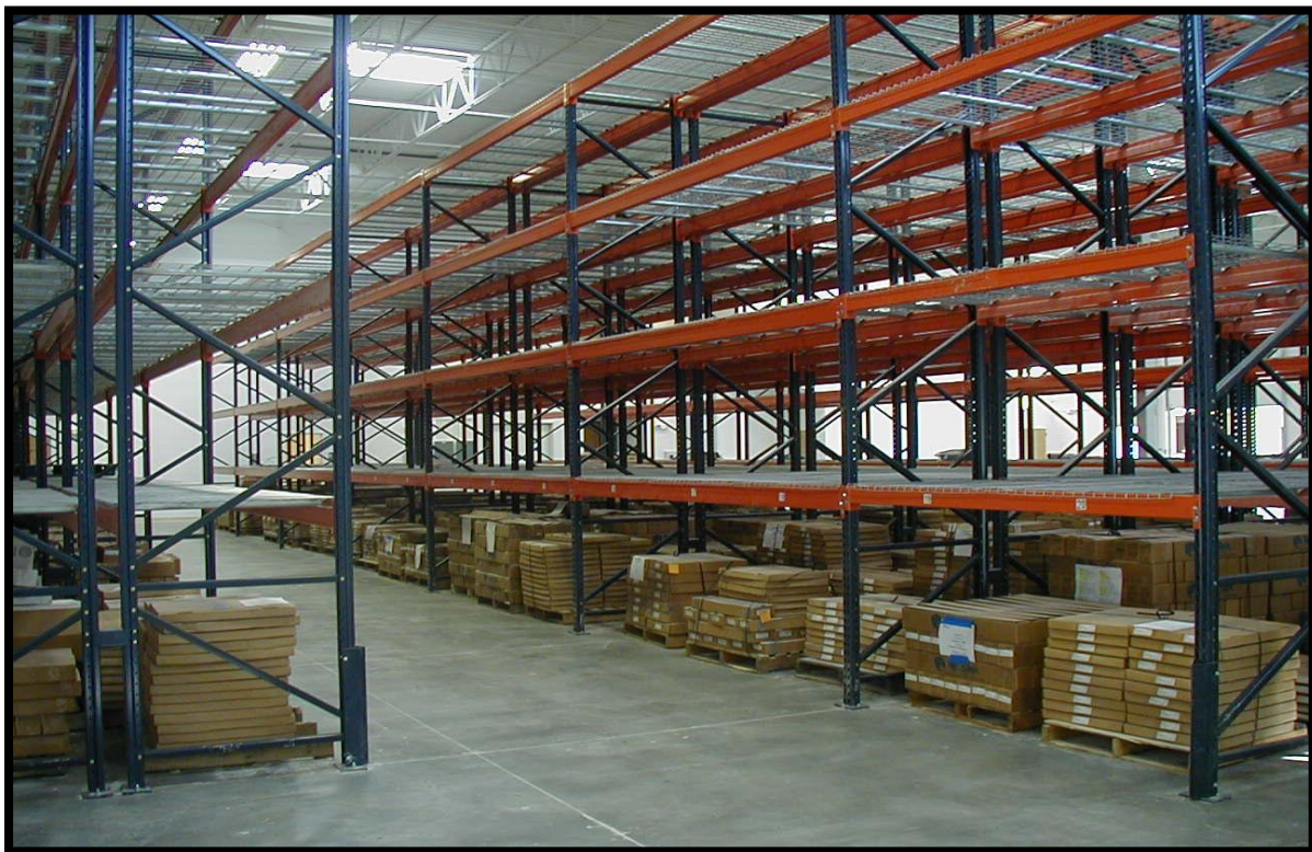
Pallet Racking: 60 Sections 16' high x 42" deep x 12' long 4 levels per section w/wire deck
